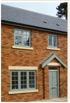
Wood Window Alliance members manufacture some of the most advanced, energy-efficient windows and doors available in the UK, whether timber or aluminium-clad. All are double or triple-glazed (with the exception of specialist period windows) and can be specified with low-emissivity glass, gas-filled glazing units and warm-edge spacer bars.
